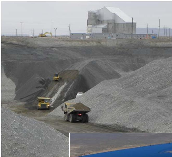
To capture the chromium plumes required uniquely engineered ramps to reach the contamination, which went 85 feet deep to groundwater.
