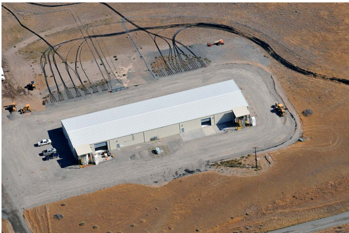
The 17,500-square-foot 100-HX process plant uses 31 extraction wells and over 61 miles of piping to bring groundwater to the facility with a capacity to treat up to 35 million gallons per month. The treated water is then returned to the aquifer through a series of injection wells.
