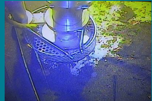
Vacuuming of solid material from the basin floor to reduce basin radioactivity, as part of the deactivation process. – January 2023
