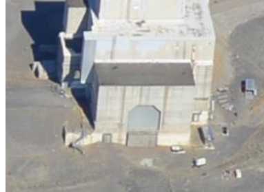
K East Reactor ready for construction of the safe secure enclosure.
