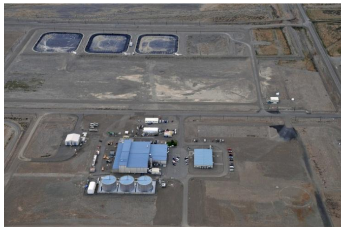
Liquid Effluent Retention Facility and 200 Area Effluent Treatment Facility
