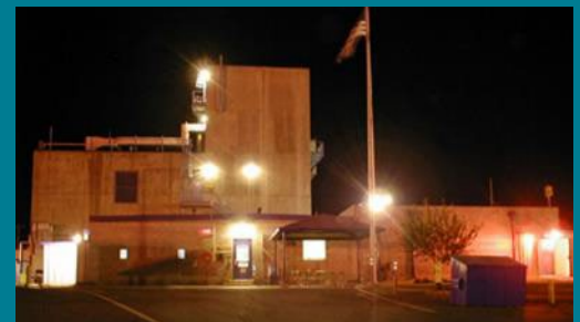
242-A Evaporator at night.
