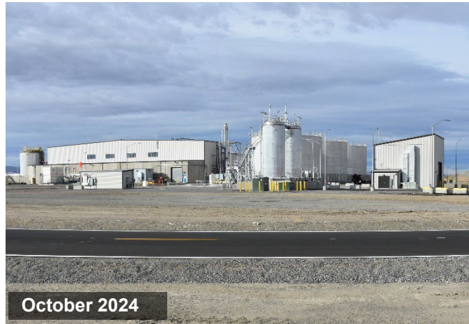
October 2024 Effluent Treatment Facility
