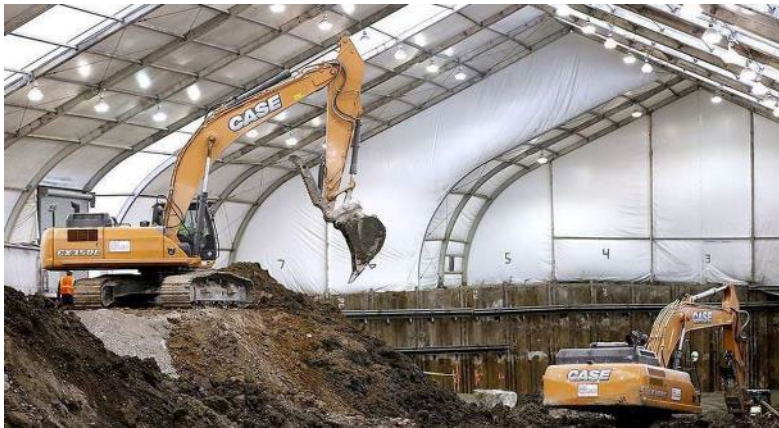
Excavation equipment inside retrieval structure
