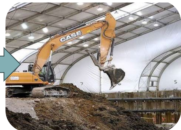
Excavation under retrieval enclosure
