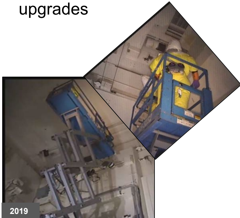
Workers use a scissor lift to repair crane equipment
