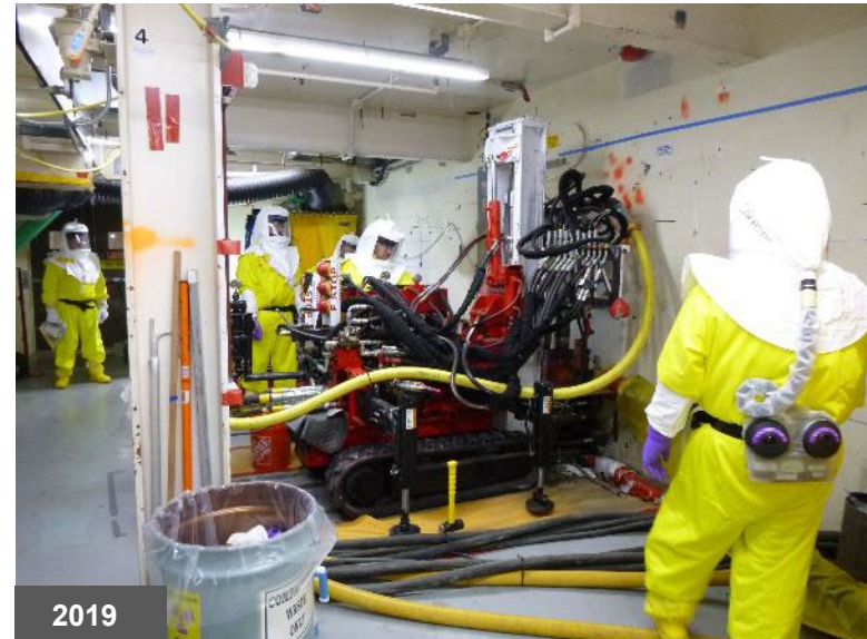
Workers operate a drill rig to support structural modifications to the 324 Building
