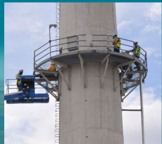
Workers conduct annual maintenance on the 324 Building ventilation stack.
