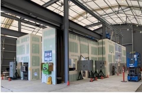
Workers constructed a mock-up to replicate features inside the 324 Building.
