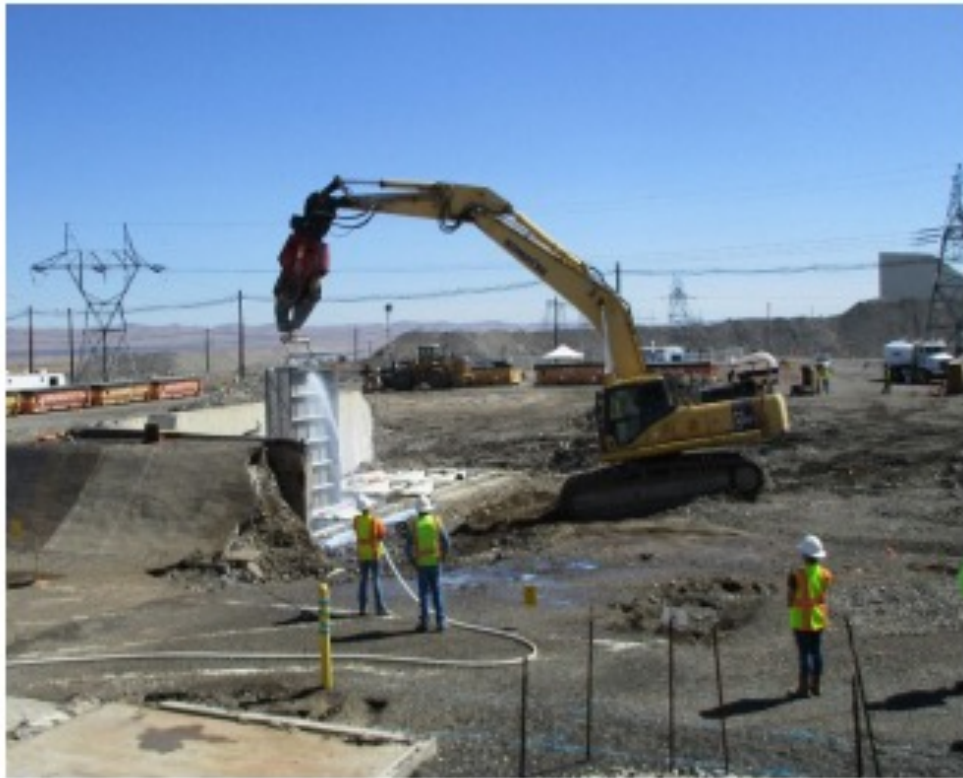
117KW Filter Removal
