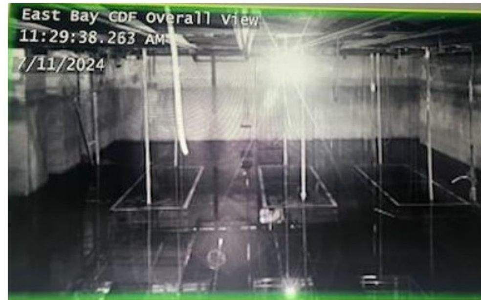
East Bay Water Removal as of July 11, 2024
