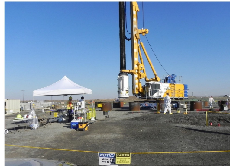
Vertical Pipe Unit Remediation
