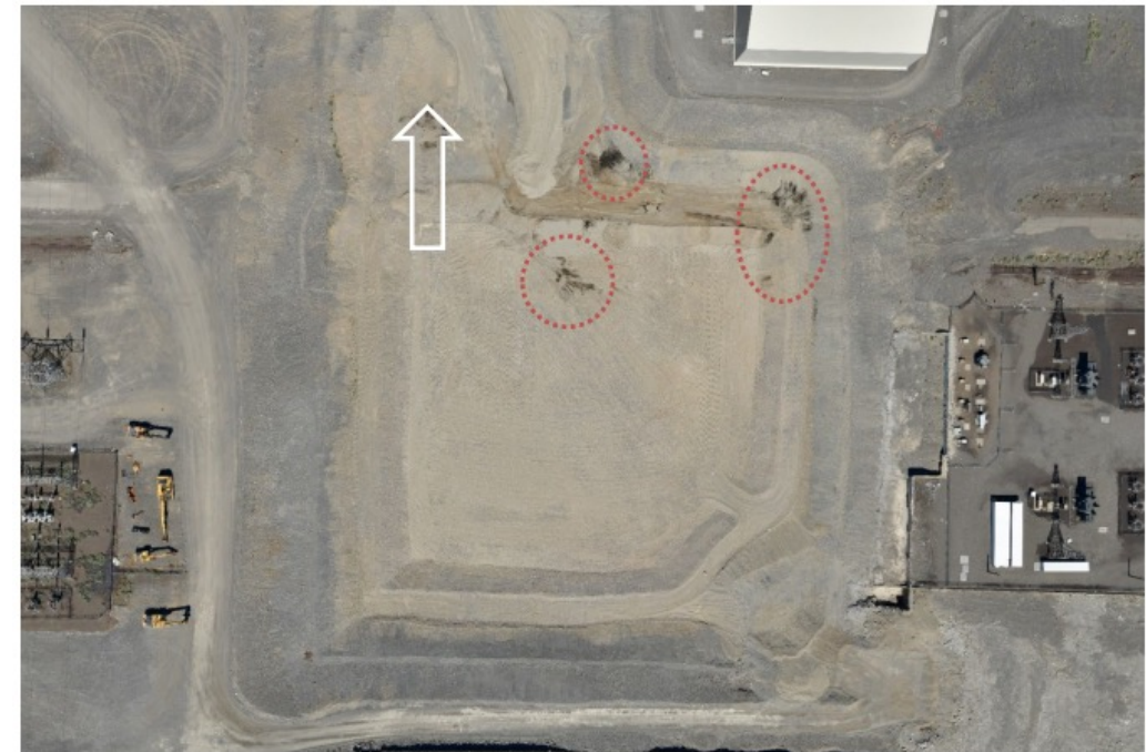
130-KE-2 Loadout of Contaminated soil to ERDF (February 2024)
