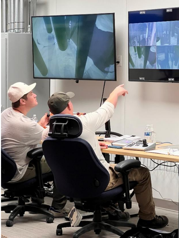
Consolidate Waste into Newer, Double-Shell Tanks
