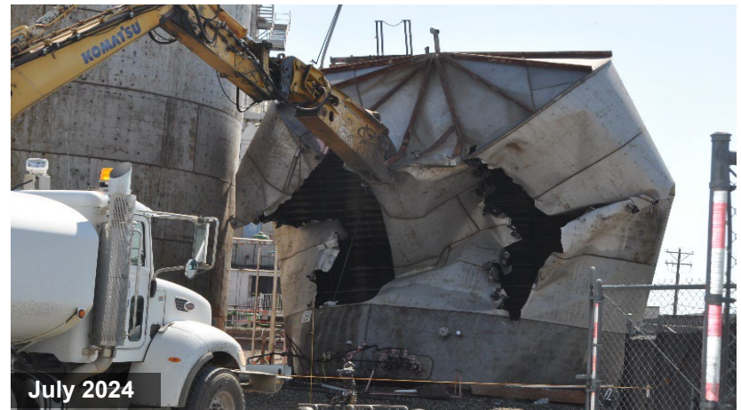
Demolition of the 211S Cold Chemical Makeup Tank Farm completed at Reduction Oxidation Plant
