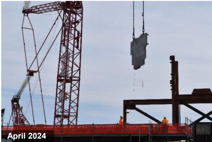
Installation of shield doors in the High-Level Waste Facility
