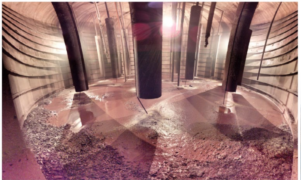
Inside Tank AX-103 after waste retrieval.
