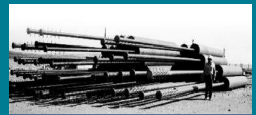
Air lift circulators before installation in waste-storage tanks. Man on right for scale.
