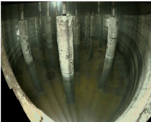
Inside Tank AX-103 before waste retrieval.
