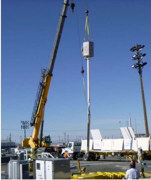
Tank AX-101 extended-reach sluice system.
