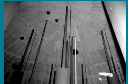
Air lift circulators in a tank. View from bottom of tank up.
