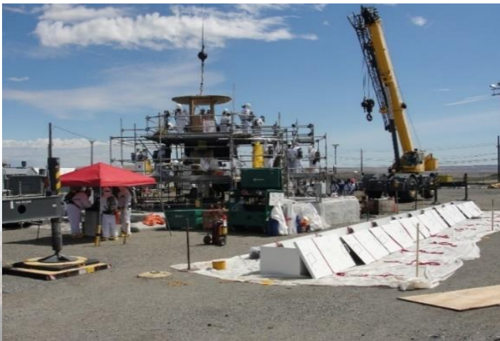
Workers removing legacy equipment from Tank A-103
