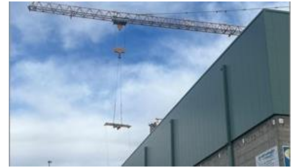
Over-the-top installation of a canister pour handling system crane
