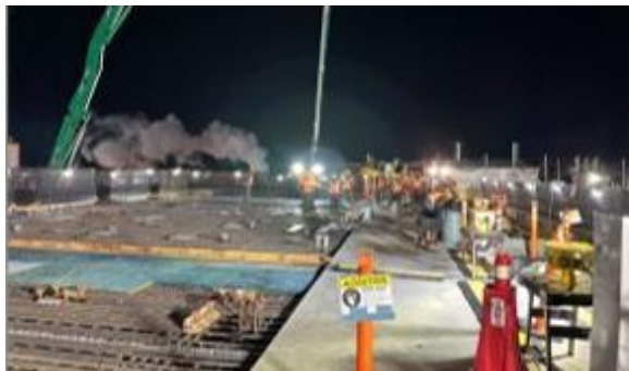
Slab placement for the High-Level Waste Facility
