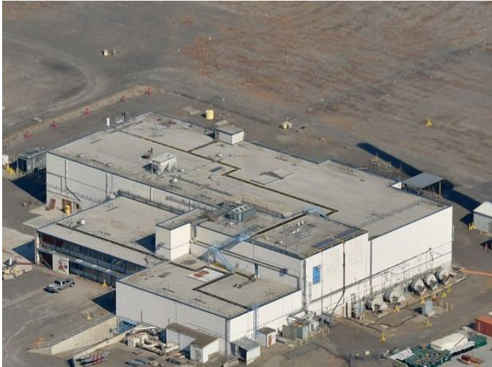
Building 324 Demolition Preparation
