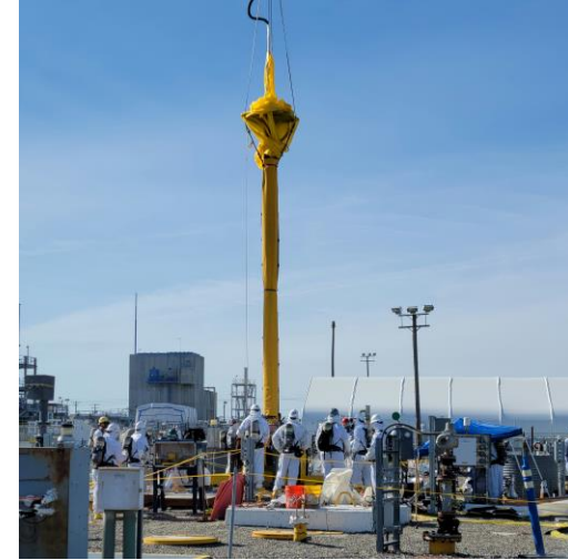
S/SX/U Tank Farm preparations
