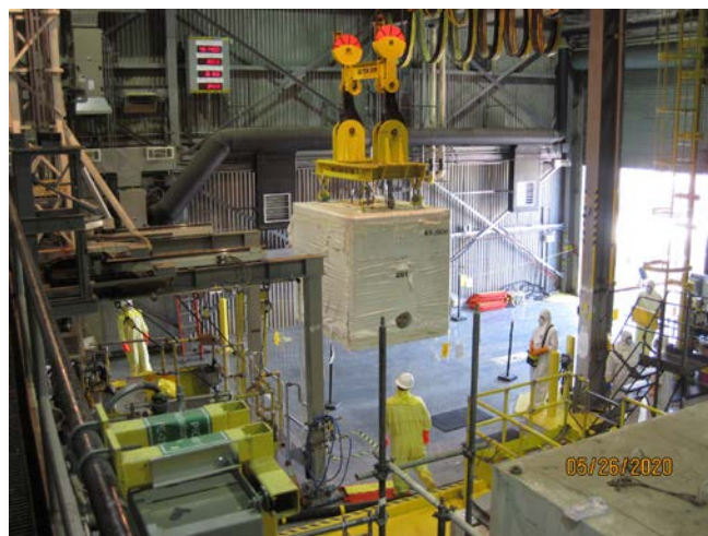
CHPRC workers replace a filter that removes radioactive cesium from water inside the 105KW Reactor fuel storage basin.
