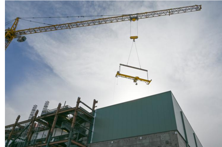
Over-the-top installation of Crane 12 into the Melter Cave #2 Support Handling System
