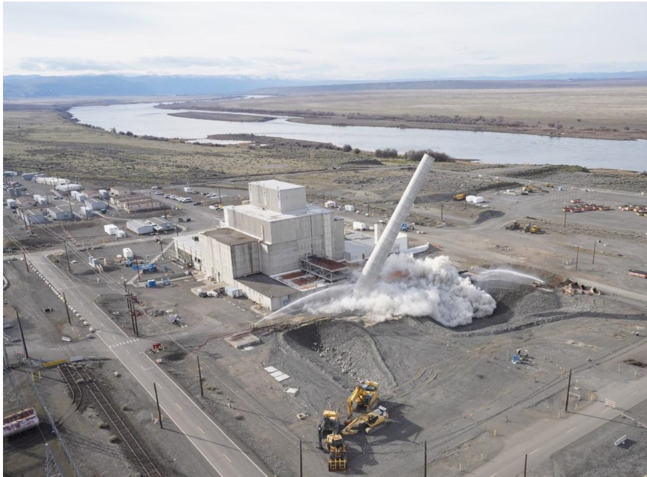
116KW stack demolition
