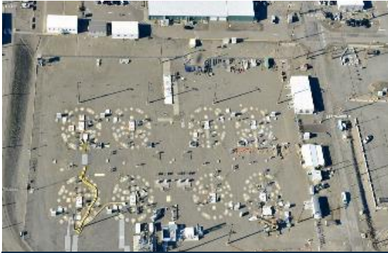
AP Tank Farm
