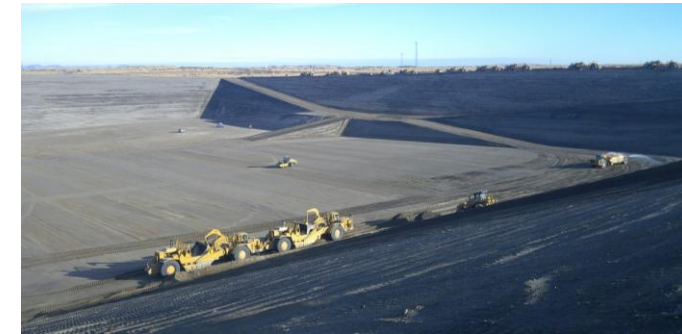
ERDF supercell excavation
