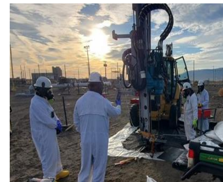
S/SX/U Tank Farm preparations
