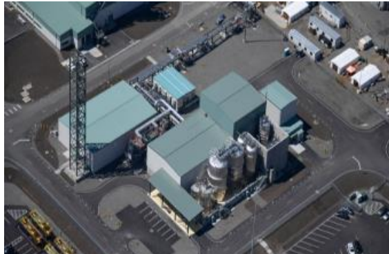
Effluent Management Facility
