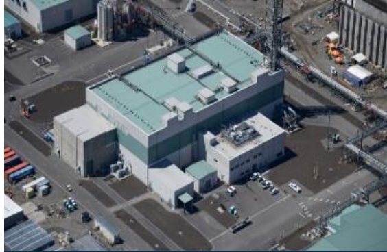
Low-Activity Waste Facility
