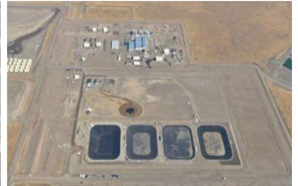
Liquid Effluent Retention Facility and Effluent Treatment Facility
