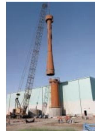
Workers guide the Canister Storage Building exhaust stack into place. The stack is part of the passive ventilation system that will use naturally circulating air to cool the spent fuel canisters.
