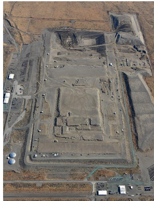
Aerial of the Environmental Restoration Disposal Facility.
