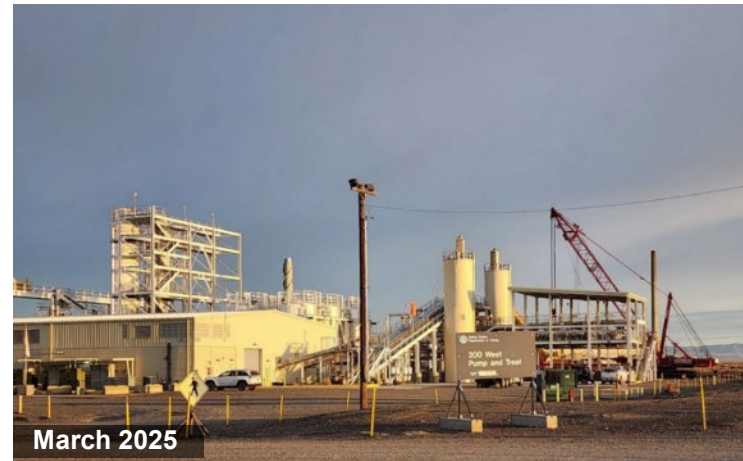
A crane is staged to install an Air Stripper Tower at the 200 West Pump and Treat Facility
