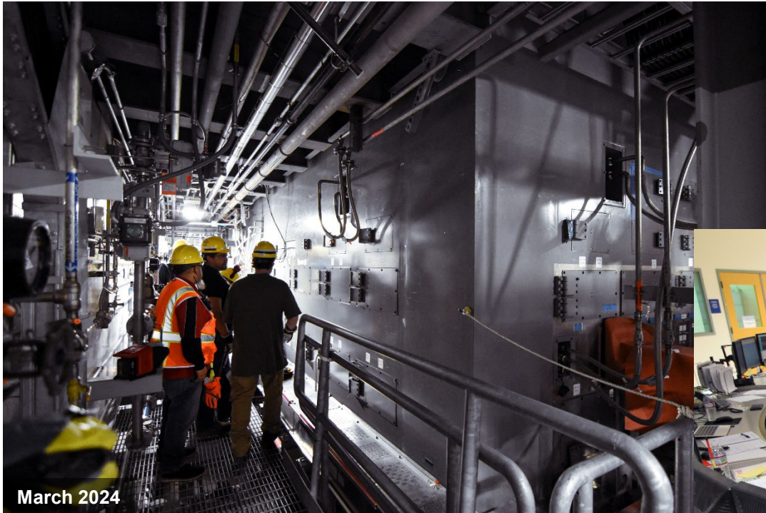
Waste Treatment and Immobilization Plant (WTP) personnel inspect the exterior of Melter 2 during the heatup process.
