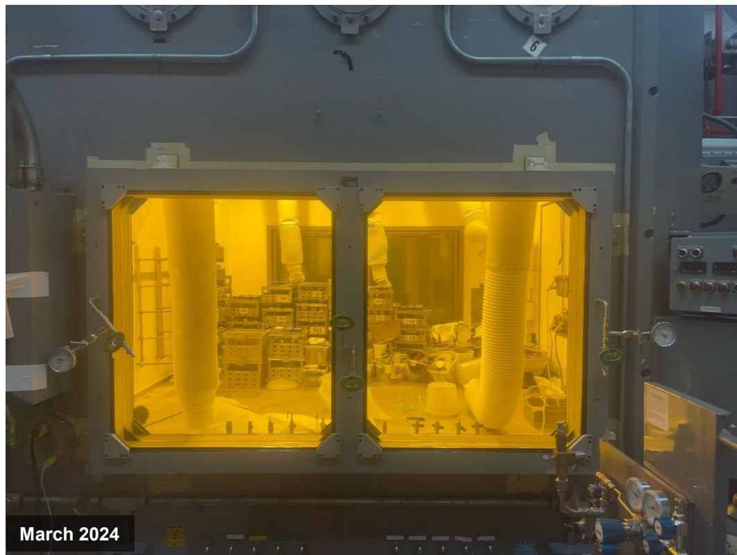
Crews removed old glass windows from Hanford's 222-S Laboratory 11A hot cell and replace them with new windows.
