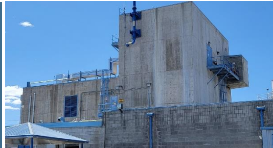
Rear view of the 242-A Evaporator in the 200 East Area
