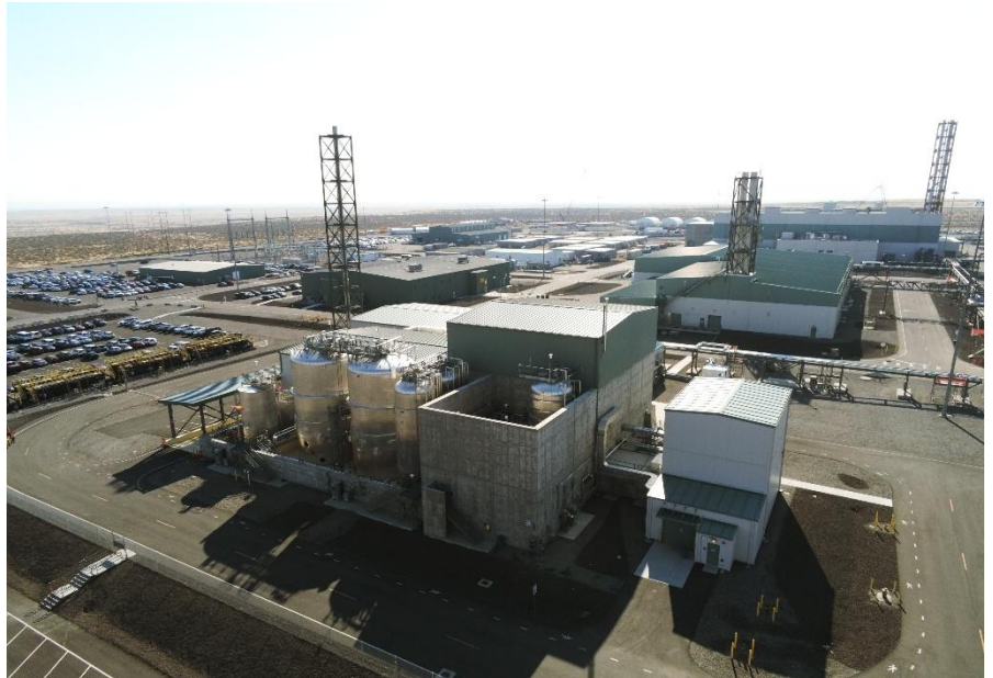
Effluent Management Facility at the Waste Treatment and Immobilization Plant
