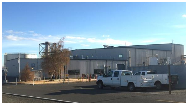
Outside the 200 Area Effluent Treatment Facility
