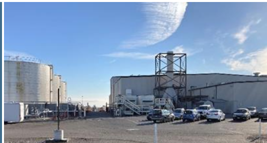
Outside the Effluent Treatment Facility
