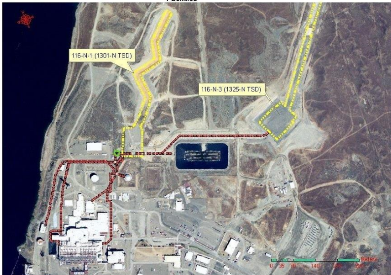
116-N-1 (1301-N) and 116-N-3 (1325-N) Liquid Waste Disposal Facilities
