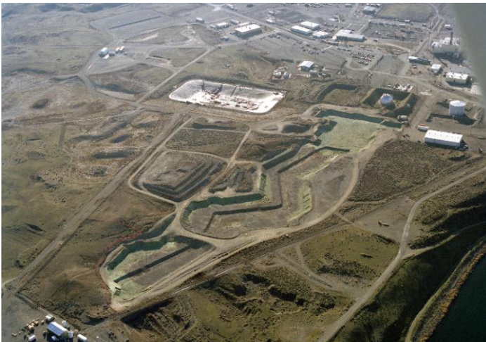
1301-N after Remediation with land Bridge for ongoing work.
