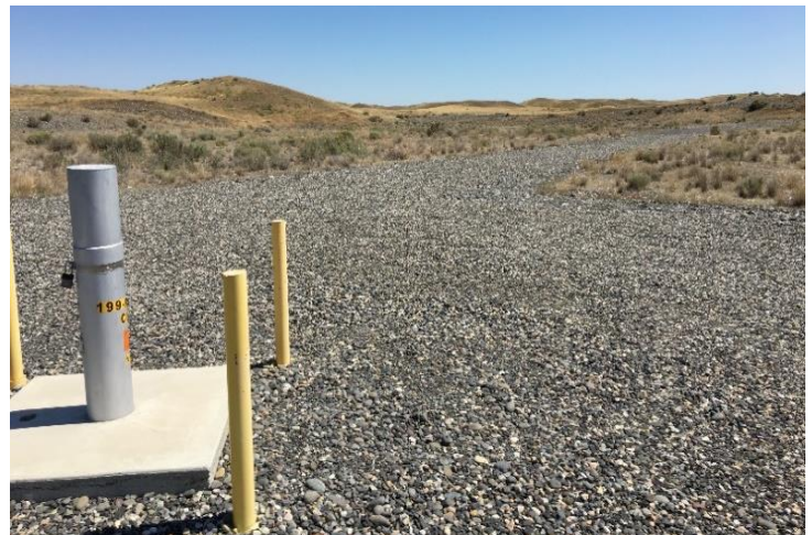
Monitoring well 199-N-188 1325-N Crib after remediation.
