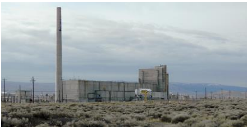
The REDOX Plant is located on the Hanford Site in eastern Washington State
