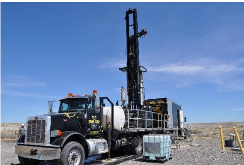
Well-drilling on Hanford's Central Plateau.
