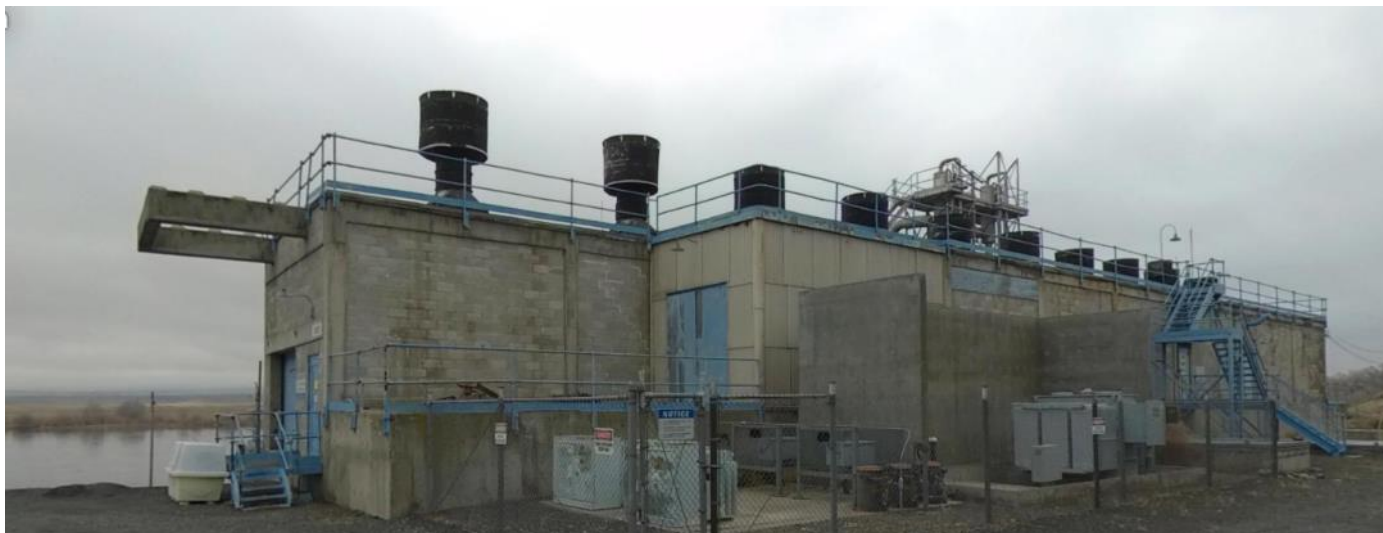
Hanford's pump stations date back to the 1940s. Work is underway to upgrade the export water system.
