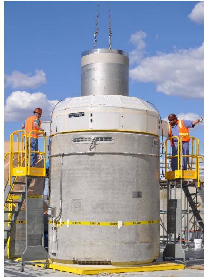
Workers are preparing to move 1,936 radioactive capsules from the Waste Encapsulation and Storage Facility to safer, dry storage.
