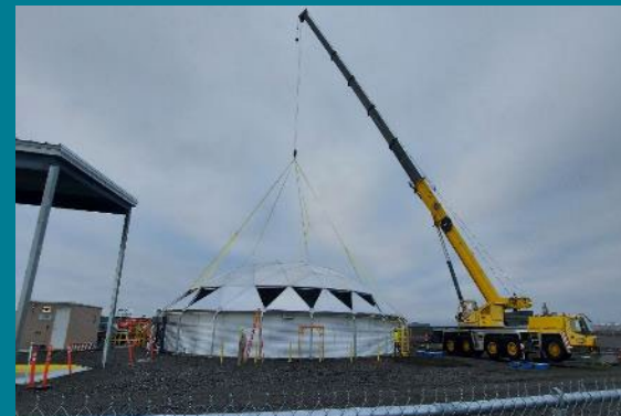
Drainage system tank domes were installed in January 2023.
