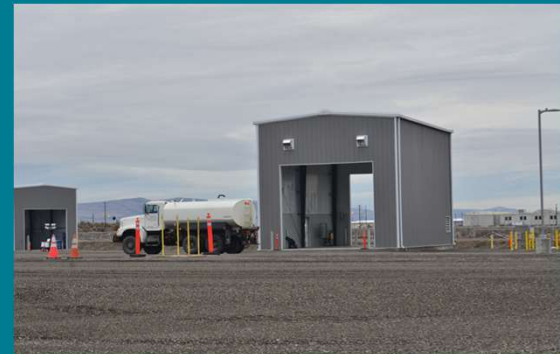
Pallet and immobilized low-activity waste transporter inspection buildings.
