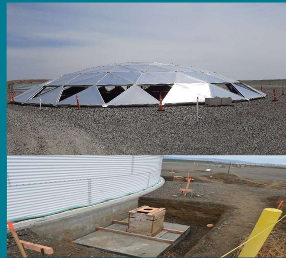
Leachate system upgrades to include dome covers, piping and structural supports.
