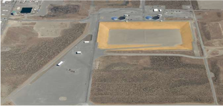
The U.S. Department of Energy and contractor Central Plateau Cleanup Company are preparing the Integrated Disposal Facility at the Hanford Site in southeastern Washington state to receive vitrified (immobilized in glass) low-activity tank waste and mixed low-level waste from Hanford Site operations.
