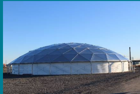
The Integrated Disposal Facility includes two 400,000-gallon tanks to collect potentially contaminated water from rain and dust-suppression activities.
