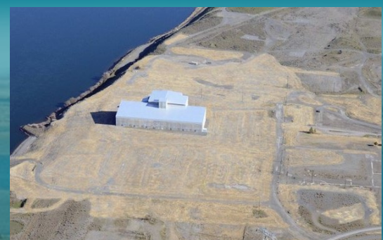
N Reactor in 2015, after Interim Safe Storage.
