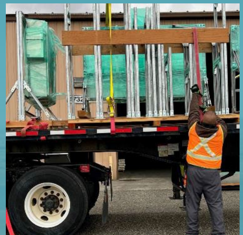
Equipment for the 2,000-gallon Test Bed Initiative demonstration is moved for modifications ahead of installation.
