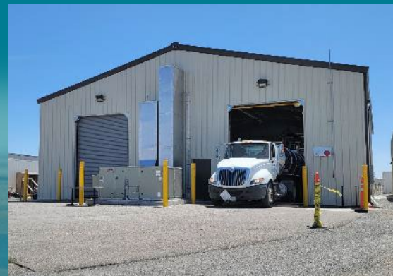
The Effluent Treatment Facility load-in building will enhance facility throughput during direct-feed low-activity waste operations.
