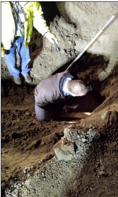
Repair of broken water line in 200 West area
