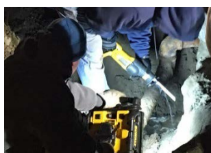
Excavation/repair of broken water line
