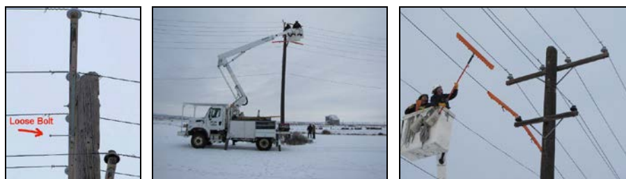
Repair of loose crossarm brace on electrical line
