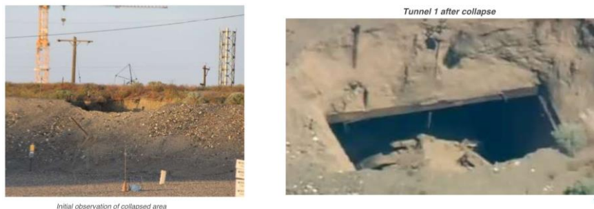
Figure 3 - PUREX Tunnel 1 collapse area (May 2017)
