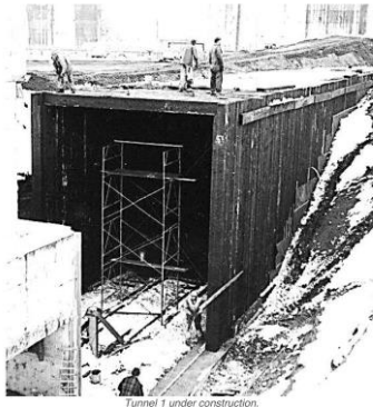
Figure 1 - PUREX Tunnel 1 under construction (circa 1956)
