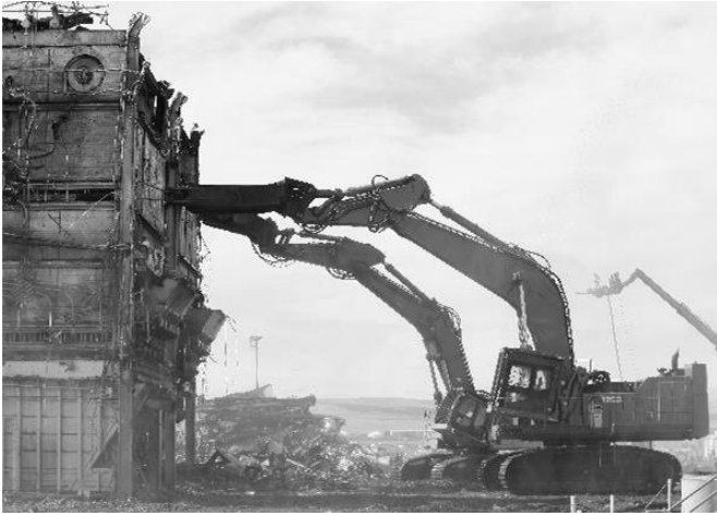
Employees successfully and safely demolished the 284 west boiler.
