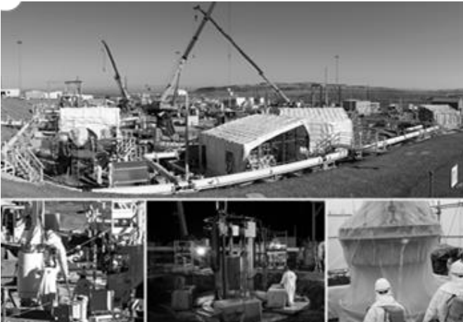
Employees handled the retrieval of C Farm tanks.
