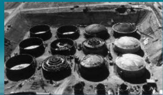
Tank Farms under construction.
