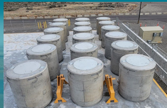
Concrete casks designed to hold cesium and strontium capsules are staged on an interim dry-storage pad.
