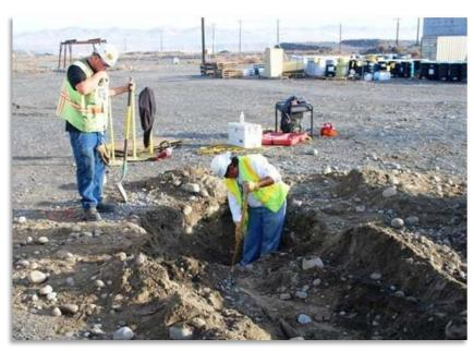
Workers dig a footing for the DX groundwater treatment facility. The facility, located in the 100 Area, is being constructed with Recovery Act funds to advance efforts to protect the Columbia River by treating hexavalent chromium contamination in the groundwater.
