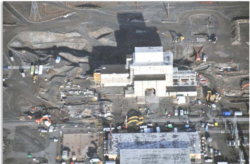
105KE Demolition Progress and 1706KE Below-Grade Demolition
