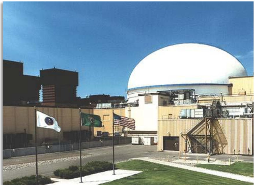
Fast Flux Test Facility
