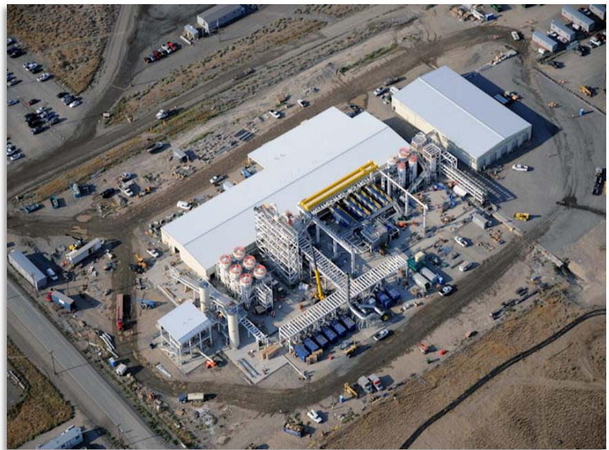
200 West Groundwater Treatment Facility – Construction Complete KPP completed on September 26, 2011
