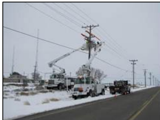
Installation of new capacitor banks in 200 West Area
