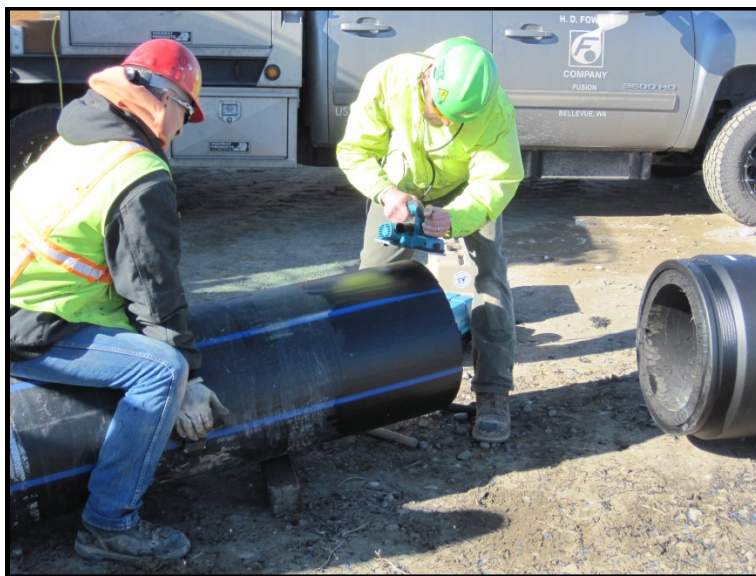
Project Z-094 – Repair of Broken Export Water Line in the 200 East Area
