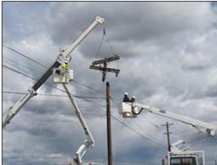
MSA Electrical Utilities personnel remove a burnt power pole
