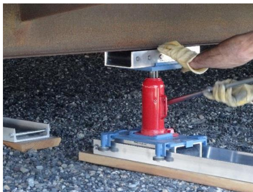
MSA Maintenance personnel use a newly acquired sliding jack system
