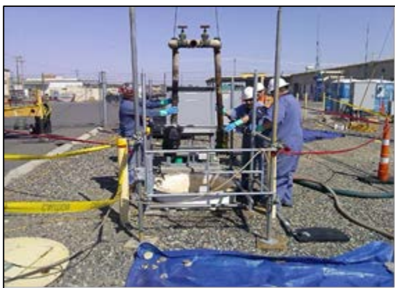
Workers Lift Old Equipment Out of 350 Building Sewer Lift Station
