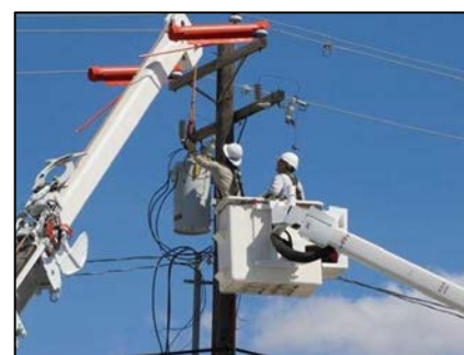
Upgrading a transformer for WRPS
