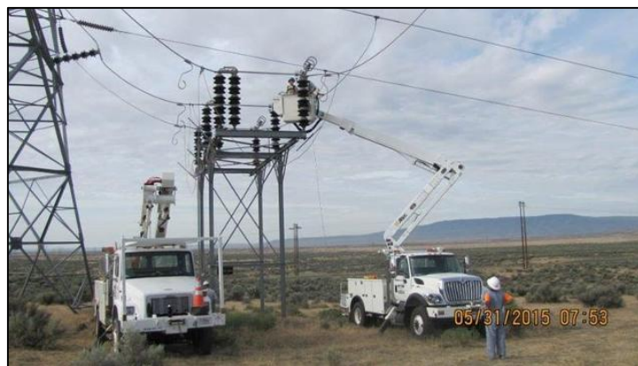
EU Crew Performing Maintenance at 230kV Ashe Tap Switching Station
