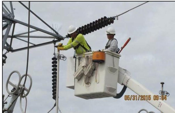
Switching Station Preventative Maintenance by Electrical Utilities Crew
