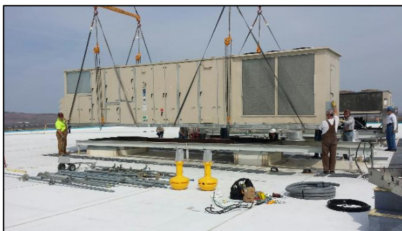
Lifting Old Unit Off the Roof of 2704HV New Unit (Left) Installed On the Roof at 2704HV
