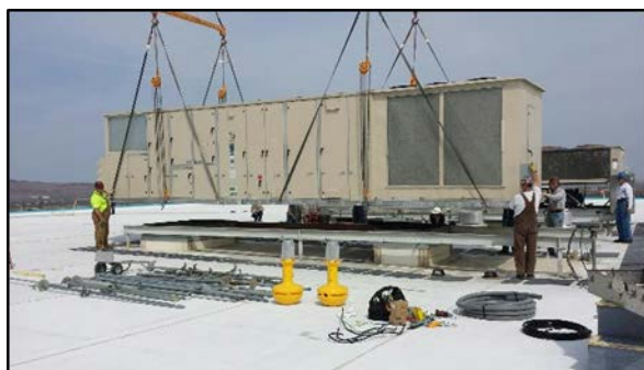
Lifting Old Unit Off of 2704HV Roof
