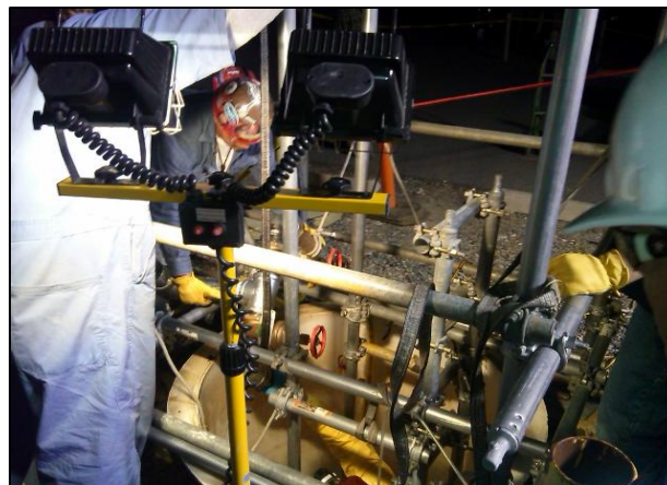
Crews Work in Confined Space to Repair Sewer Lift Station
