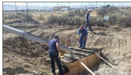
Installation of a Thrust Block after Removal of the 814 Fill Station
