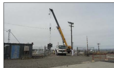
Transformer Being Loaded for Disposal
