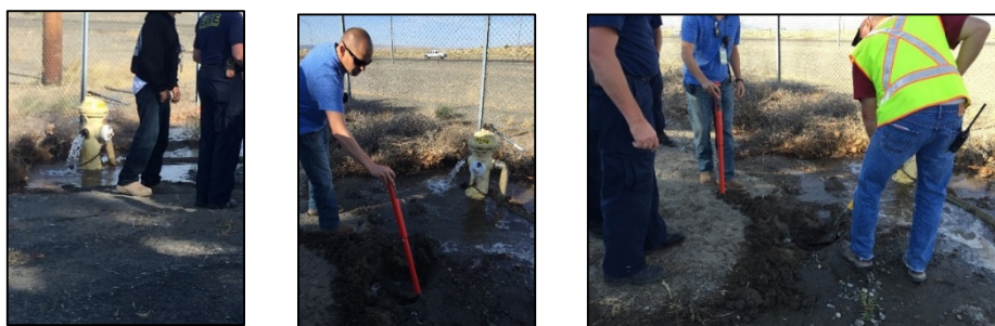
W&SU Staff Replaces Leaking Fire Hydrant Head
