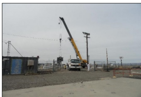
Transformer Being Loaded for Disposal
