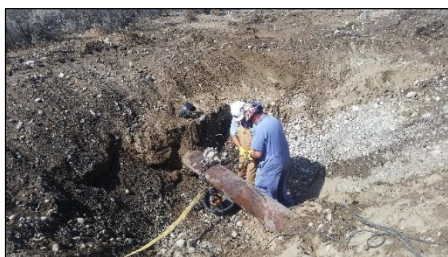
Pipefitters Cutting the Water Line to Remove the 814 Fill Station
