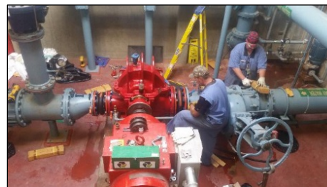
Repairing potable water fire pump
