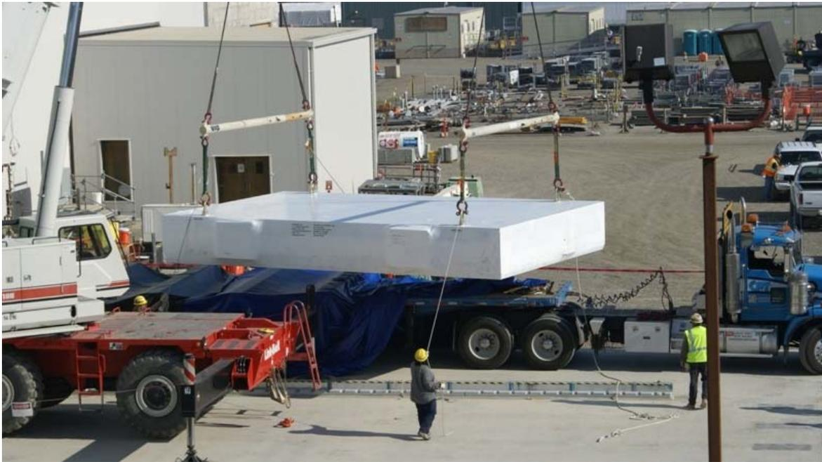
A 30-ton LAW Melter lid is off-loaded at the Waste Treatment Plant construction site.
